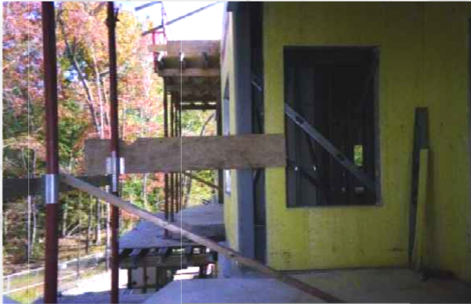
Figure 1: CIP Formwork for Balconies
