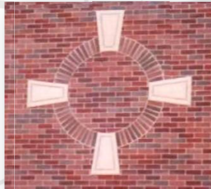
Figure 2: Thin Brick Precast Panel (API Manufacturer: www.apiprecast.com )
